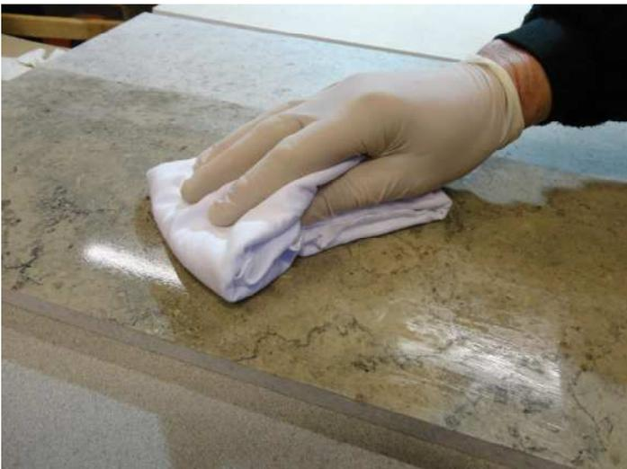
Using the same pad, even-out the remaining sealant to leave a very thin film on the surface. The aim is to leave a very light film that will 'disappear' as the sealant starts to dry. Make sure your cotton pad is dry, clean and neatly folded.
